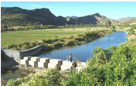
Water harvesting check-dam-Gunfel Wukro kilte awlae'lo
