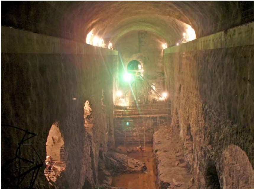
Underground powerhouse: Excavation completed view
