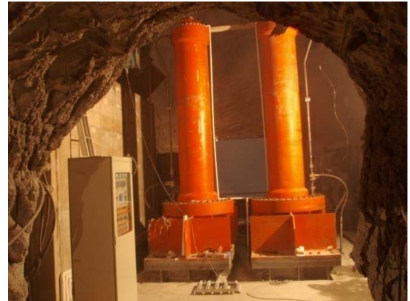
Bonnet gate HPU inside the Dam Gallery
