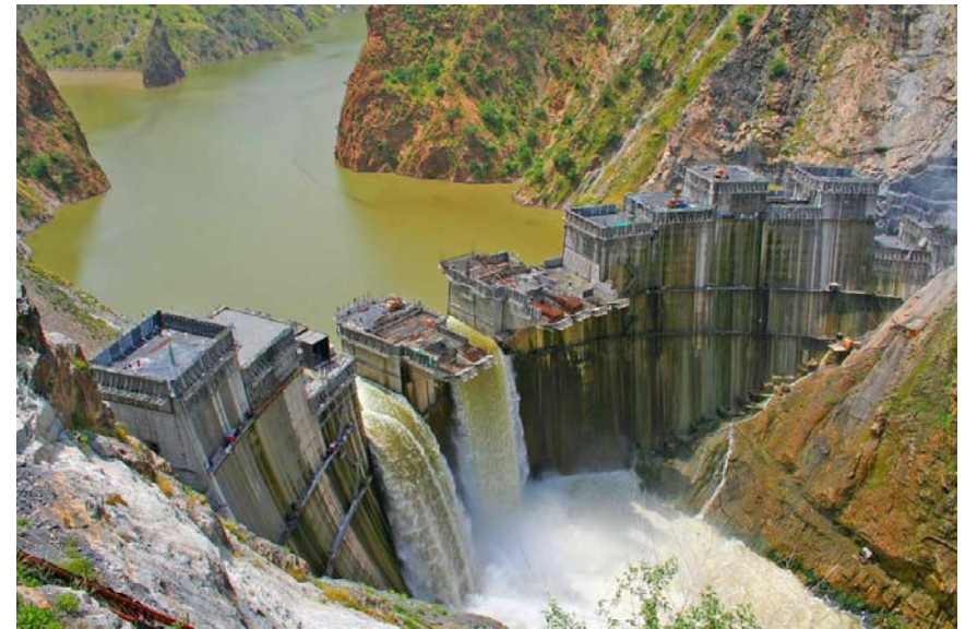
Impounding was started before the dam was completed, in order to enable generation start as early as possible
