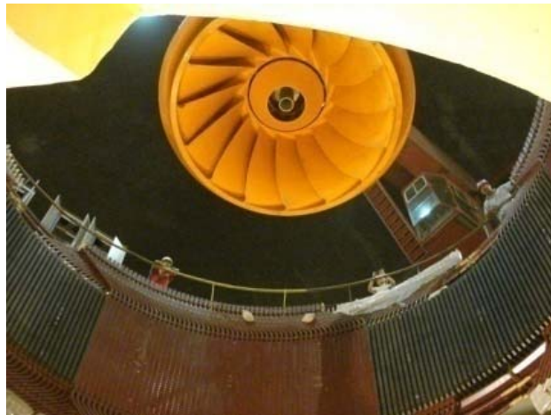
Shaft runner assembly installation
